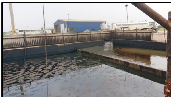
Figure 1; Hydraspin installation on the pit
