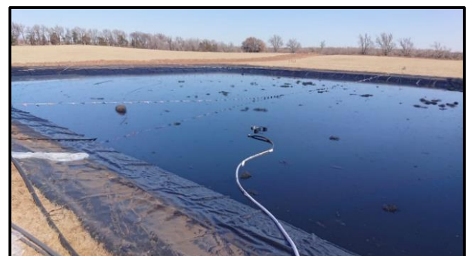
Figure 3; Hydraspin Installation other side of the dam.
