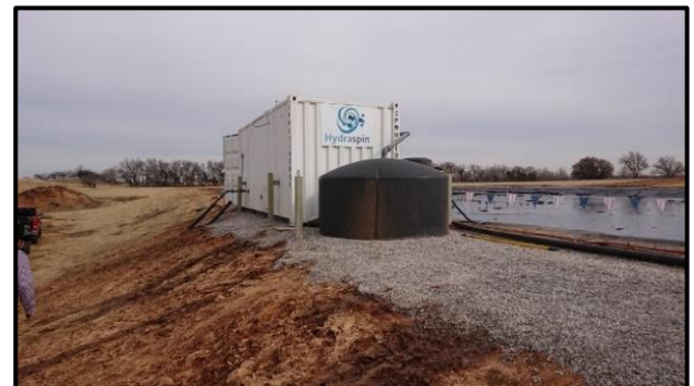
Figure 2: Hydraspin installation on a dam.
